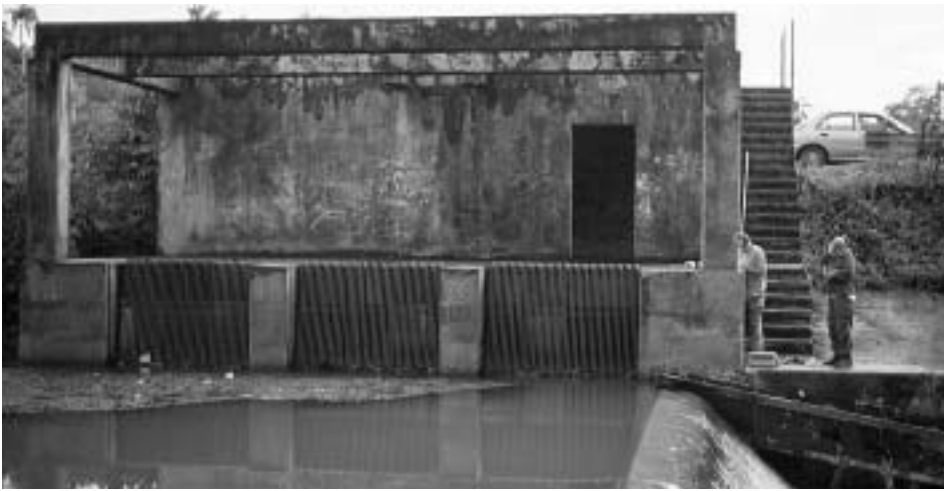
Figure 5. Fish ladder on the Río Espíritu Santo. The fish ladder is on the far right, below the people. It looks like a ramp in this photo.
